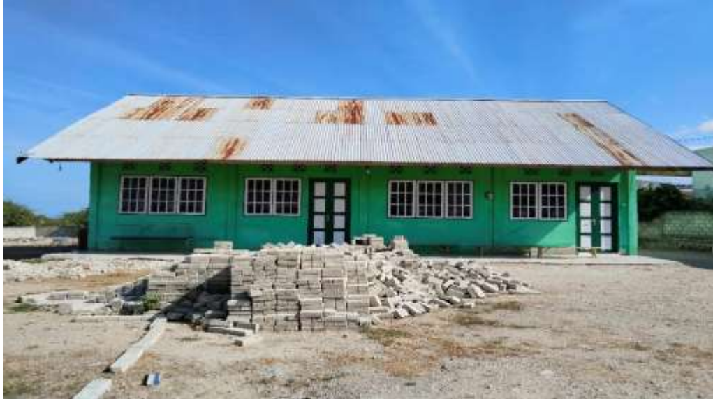
Gambar 1 Gedung TPA Nurul Khairaat
