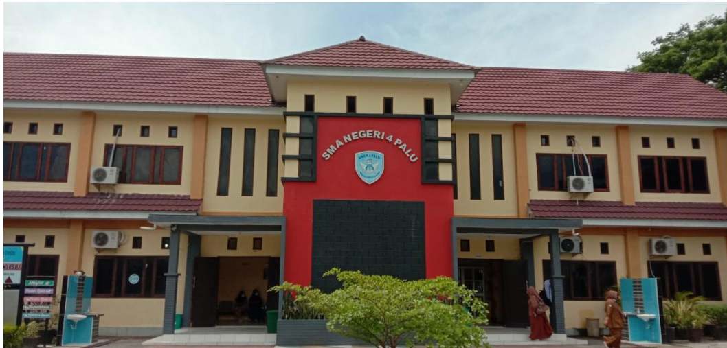
Picture 1. Front View Of SMAN 4 Palu Building
